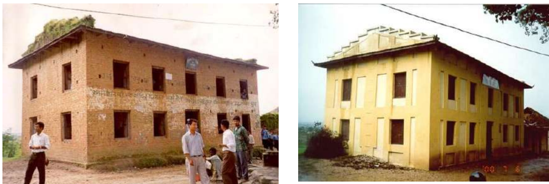
Fig. 6: Bhuaneshwori Lower Secondary School, Bhaktapur, the first retrofitted school by NSET, above pictures are of before and after retrofitting in 1997 (Source: NSET Archive)
