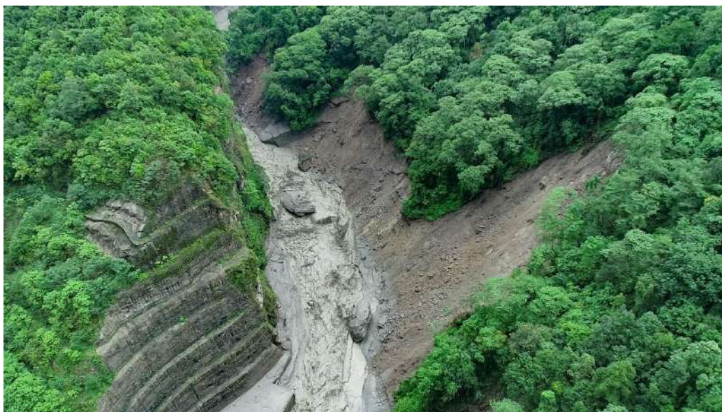
Figure 9: Big size boulders exist near the intake area of Melamchi Drinking Water Supply Project
