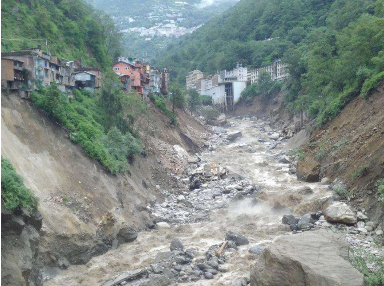
Figure 7: bank failures due to GLOF event in 2016 in Bhotekoshi River
